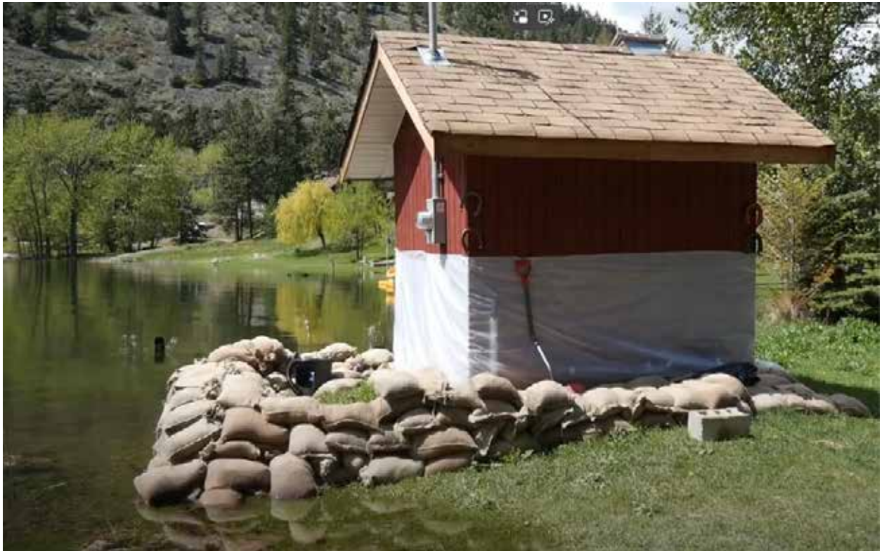
Lower Nipit well pumphouse during flood event 2021
