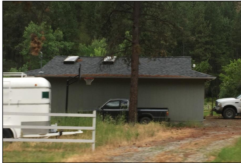
FIGURE 12 Ponderosa pine cast a considerable amount of needle litter that can accumulate on roofs and in rain gutters. The risk here is of ember ignition of the needle litter and subsequent ignition of the roof. Periodic removal is recommended to keep these hazardous fuel accumulations to a minimum.
