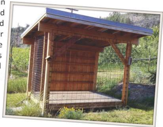
Apiary structure cost $750 in materials and labour.
